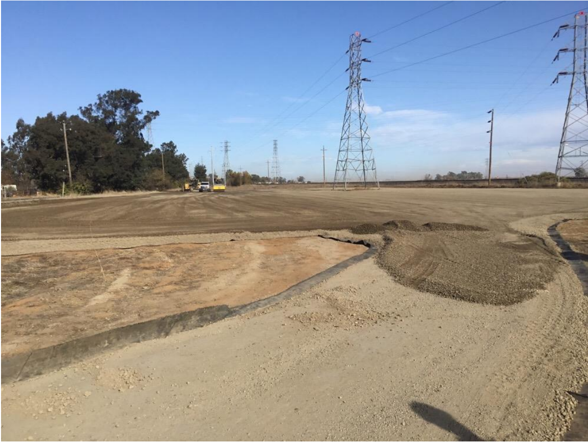
Photo 1: The CPUC EM observed winterization of Landing Zone (LZ) 40/295.
