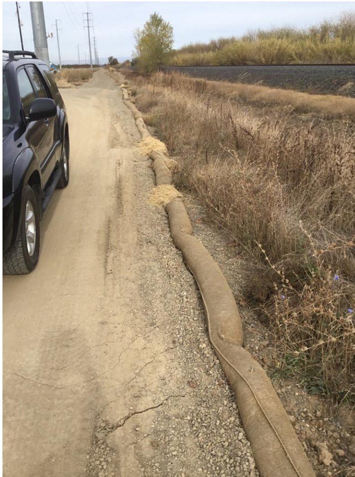
Photo 4: During routine SWPPP BMP checks, all silt fencing and wattles were found to be in good condition.
