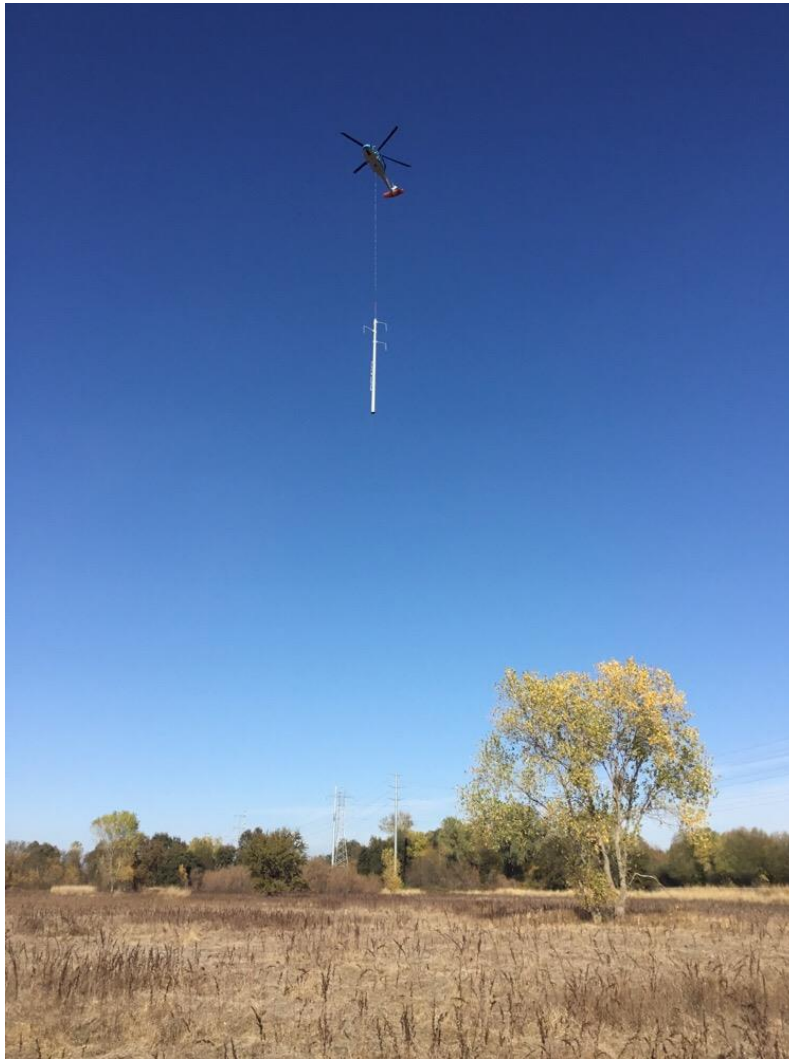
Photo 2: Helicopter observed installing a new tower top structure at site 11/87.
