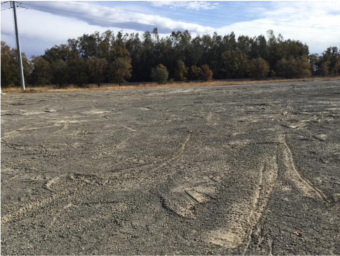
Photo 3: Old tower debris was removed from LZ 4/31 during this reporting period.
